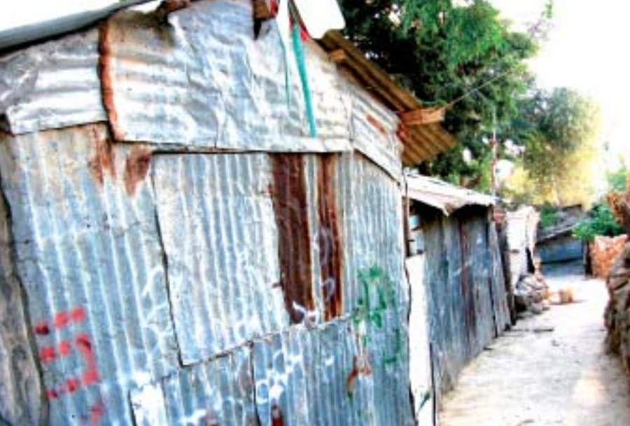
Palestinian residing in make-shift shelters with zinc roofing, Burj el-Shamali refugee camp, Lebanon, 2007. (Source: Stefan Christoff)
